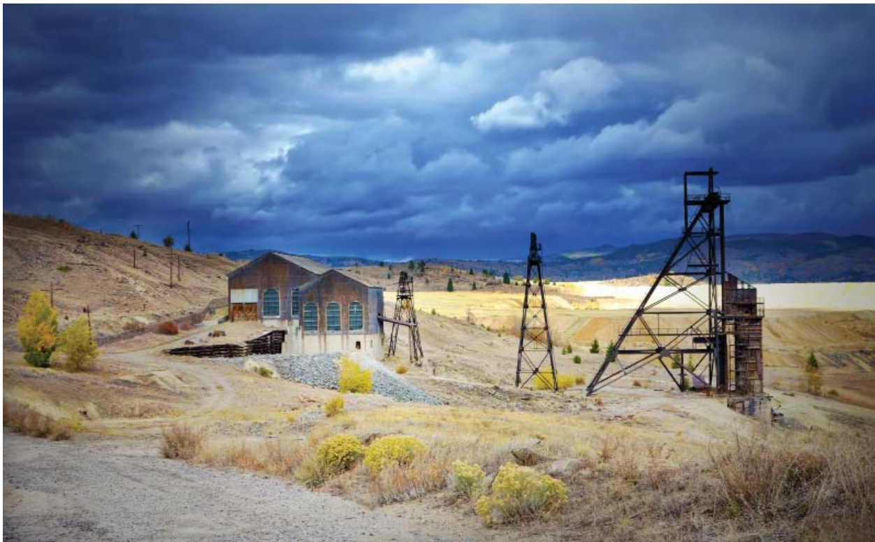
Old mine headframe in Butte, MT
